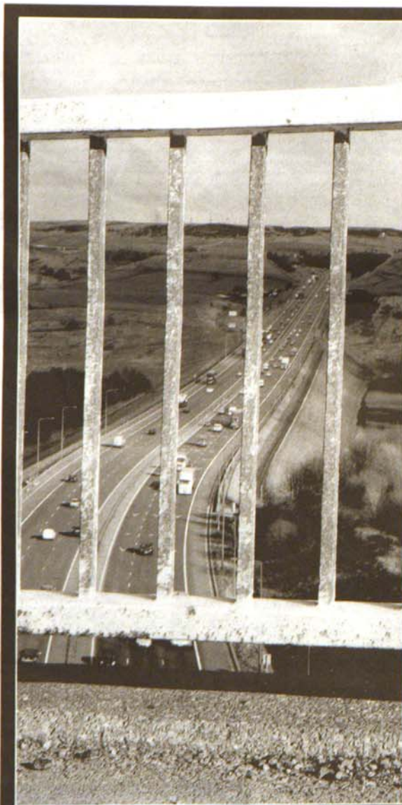
■ LAST LINE: Railings on M62 bridge at Scammonden
